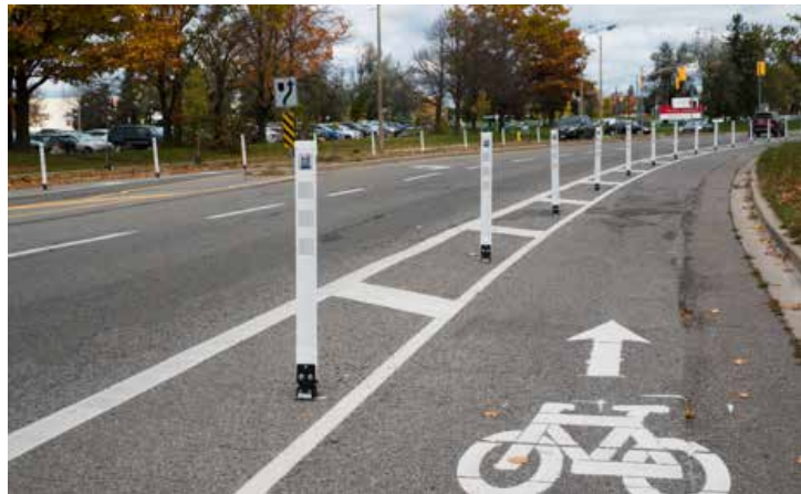
"Cyclo-Zone" Flexible Bollard - Toronto, ON (Image credit: Develotech)
