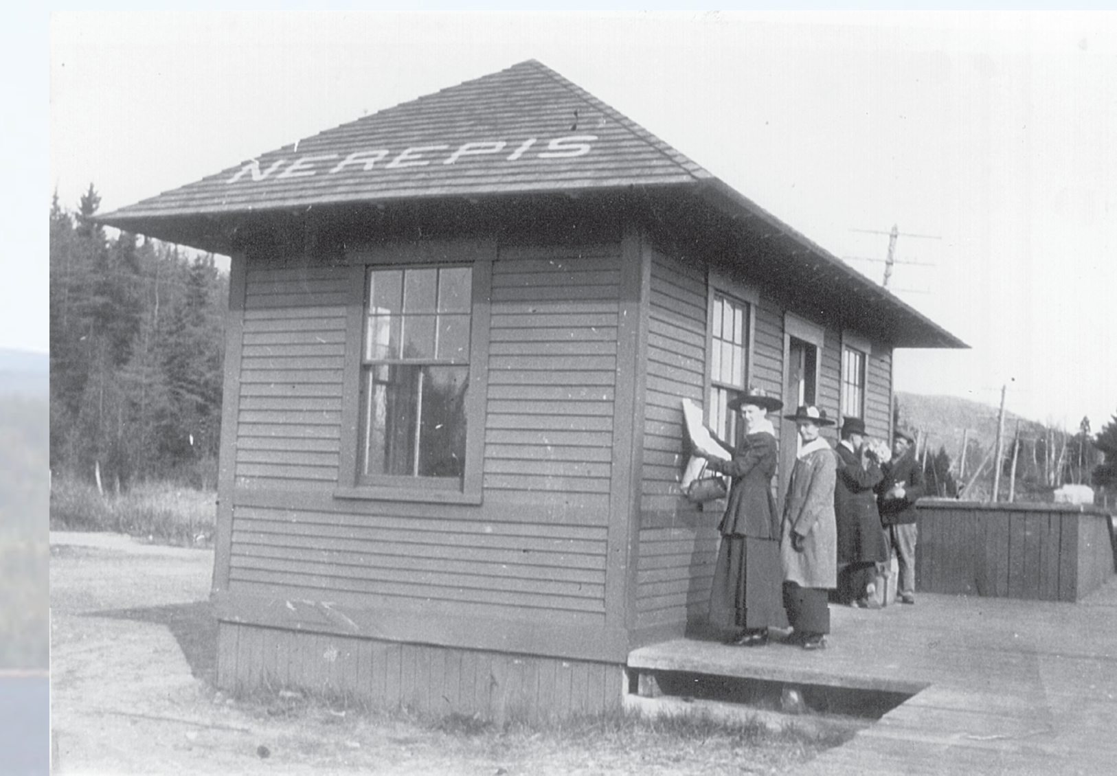
The Nerepis Station in May 1917 - located on the down river side of the Brittain Road entrance and used as a shelter.
